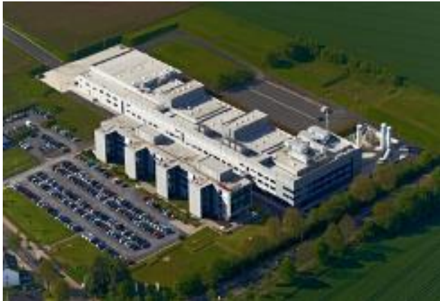
AIXTRON SE Headquarters Herzogenrath, Germany
